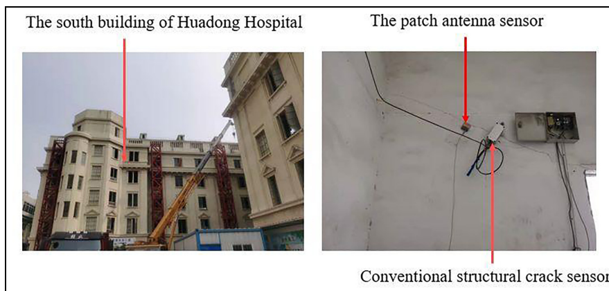
Figure 21. The building renovation project and the installed patch antenna sensor.
