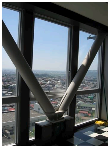
Fig. 4. Oil damper brace.
