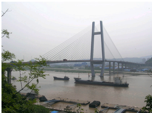
(a) Photo of target bridge
