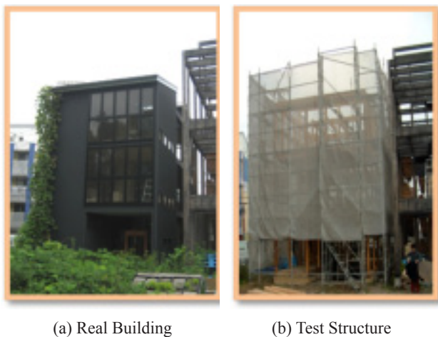
Fig.1. Test Structure On-site
