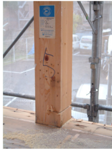
(a) Half-cutting at column-base (HC)
