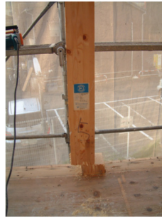
(b) Full-cutting at column-base (FC)
