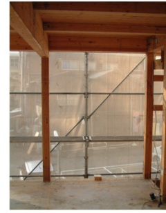
(c) Removal of column (RM)
