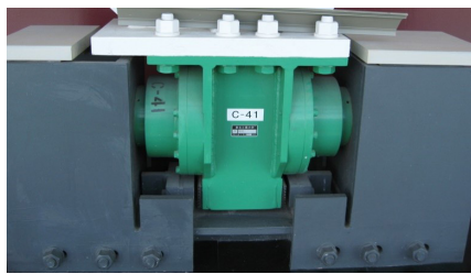
Fig.4. Intact Oil Damper
