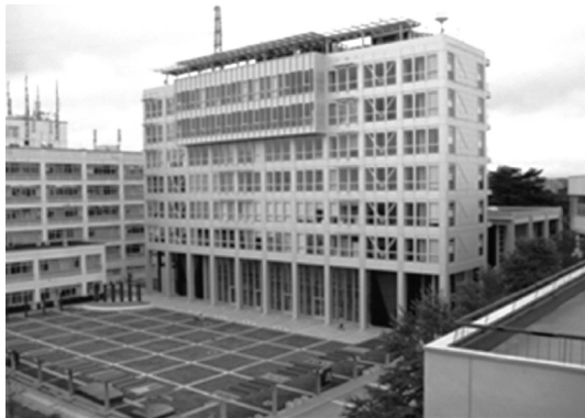
图 1 位于日本仙台的油阻尼器钢结构行政楼 Fig.1 Administration building with oil dampers in Sendai City, Japan
